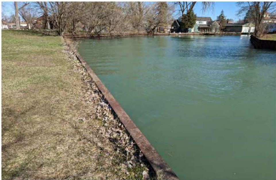
PHOTO 2: TREES BEHIND NORTH SEAWALL
