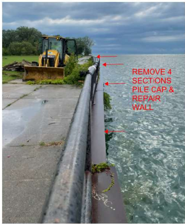
PHOTO 2: LOOKING WEST ALONG SEAWALL
