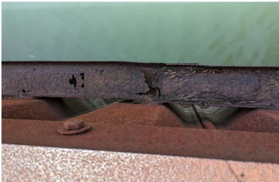
PHOTO 3: DETERIORATED WALER
